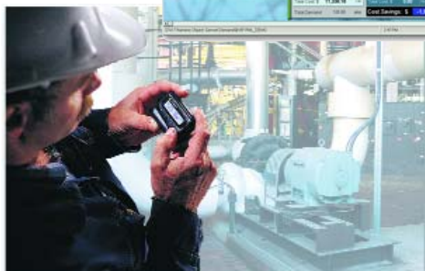
Receive alarms via pager or email. Automatically control the operation of boilers, generators, or other equipment.
